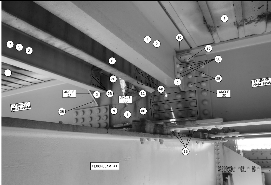
VIEW LOOKING EAST FROM THE SOUTH FACE OF FLOORBEAM 44
