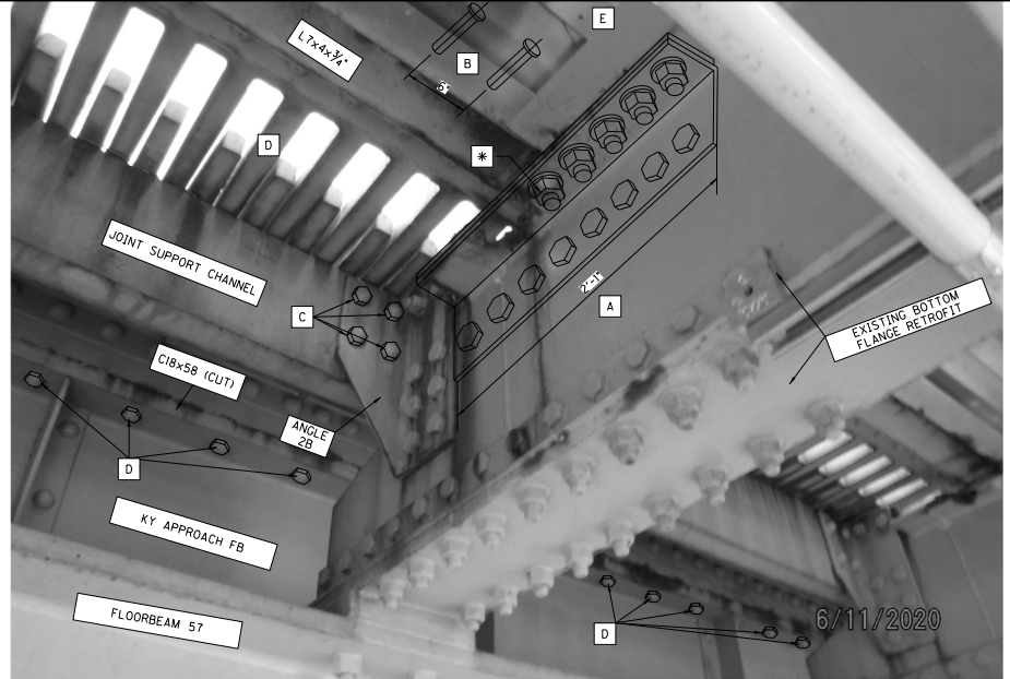
LOOKING SOUTHWEST FROM THE NORTH FACE OF FLOORBEAM 57
